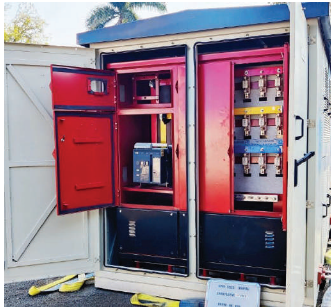
Fig. 4 : Low voltage switchgear and controlgear compartment
