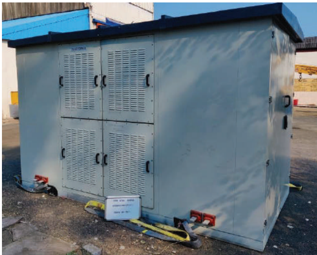
Fig. 2 : External layout of compact substation
