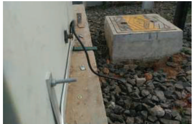
Fig. 4 : Vertical pipe earth electrode .
